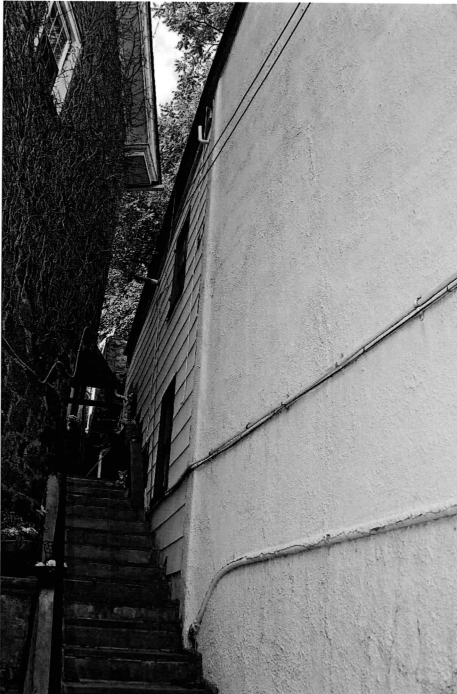
Photo 4 of 14: West elevation, addition. 9/8/2016
