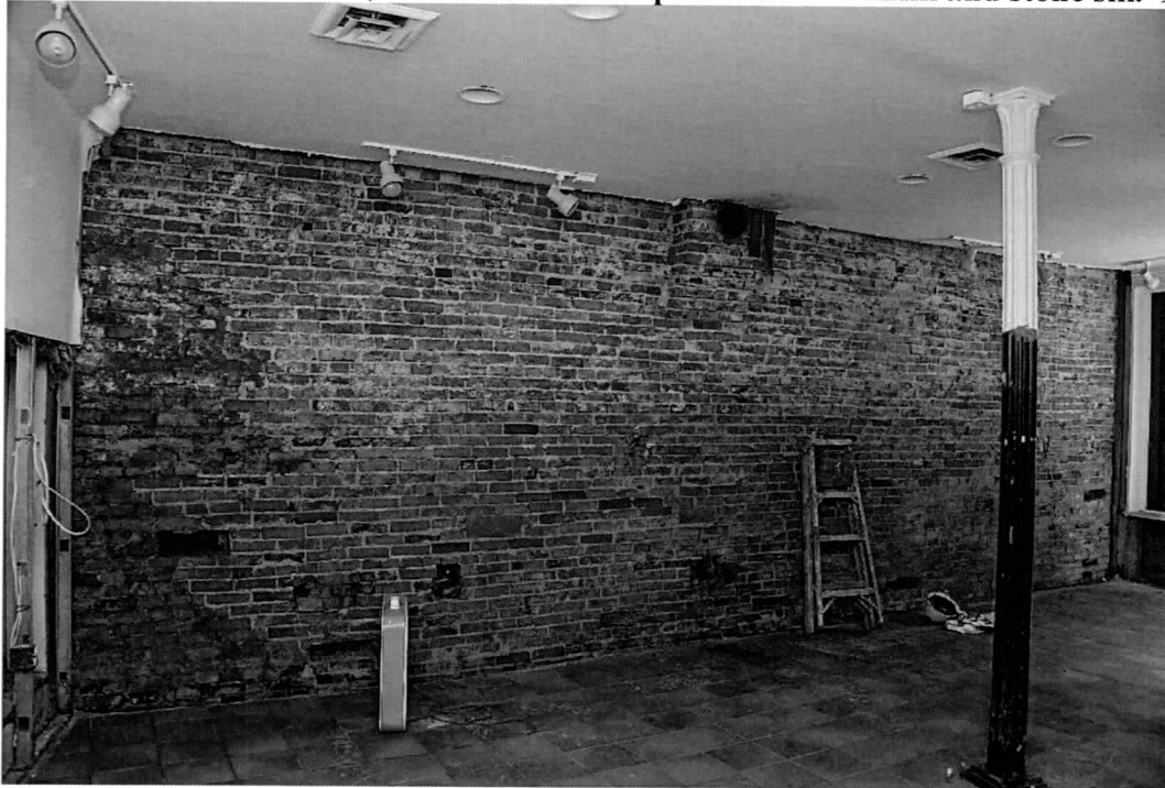
Photo 9 of 14: Basement, east wall. 9/8/2016
