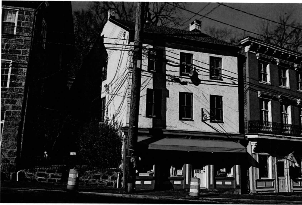
Photo 1 of 14: West & south elevations. 2/23/2021
