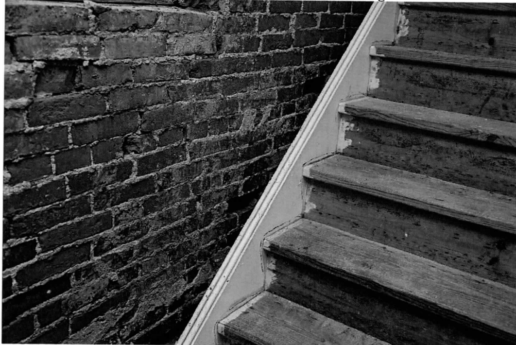
Photo 11 of 14: Basement, west wall showing nailing block holes behind existing stair. 9/8/2016
