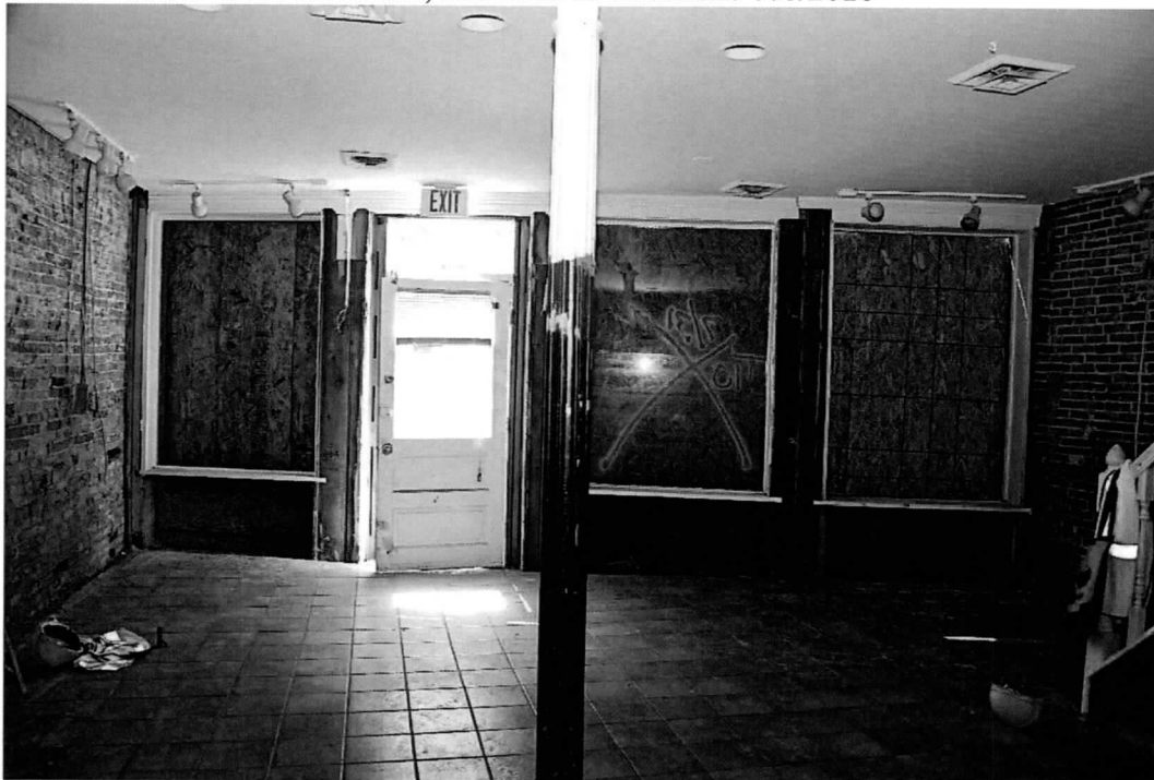
Photo 7 of 14: Basement, south wall. 9/8/2016
