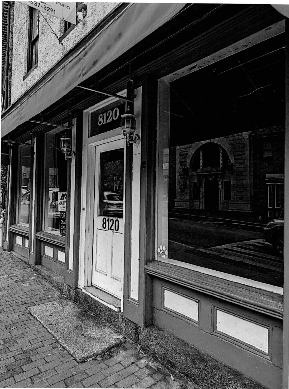
Photo 3 of 14: South elevation, storefront. 11/15/2024
