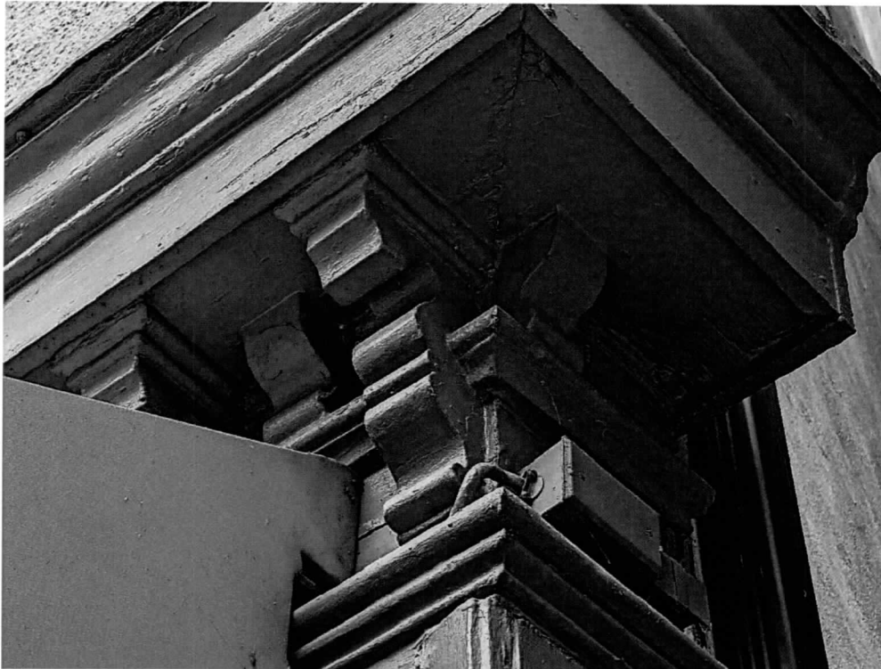
Photo 2 of 14: South elevation, storefront cornice. 11/15/2024
