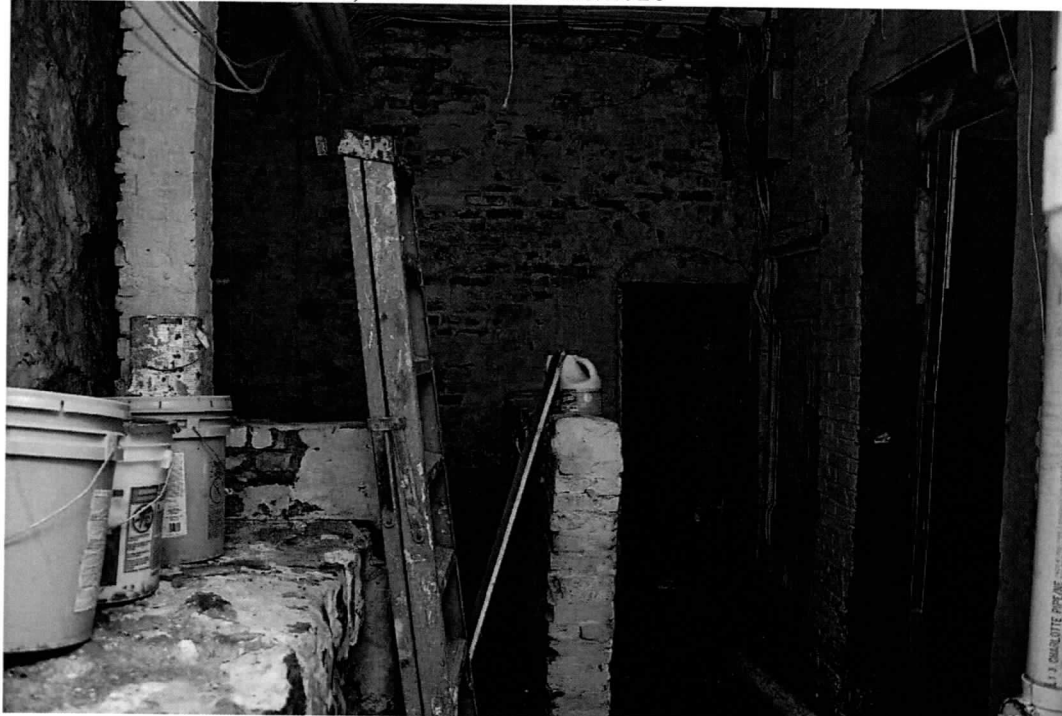
Photo 14 of 14: Basement, below addition, view east. 9/8/2016
